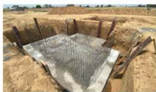
600 MW Jhansi Solar Park: Work of Internal Power Evacuation is under Progress
