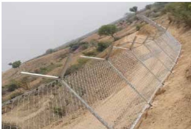
Fencing Work at Jhansi Solar Power Park
